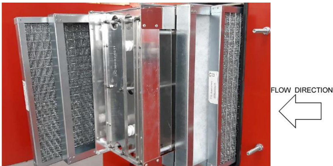
Photo No.3 – Placement sequence of the filtration elements
