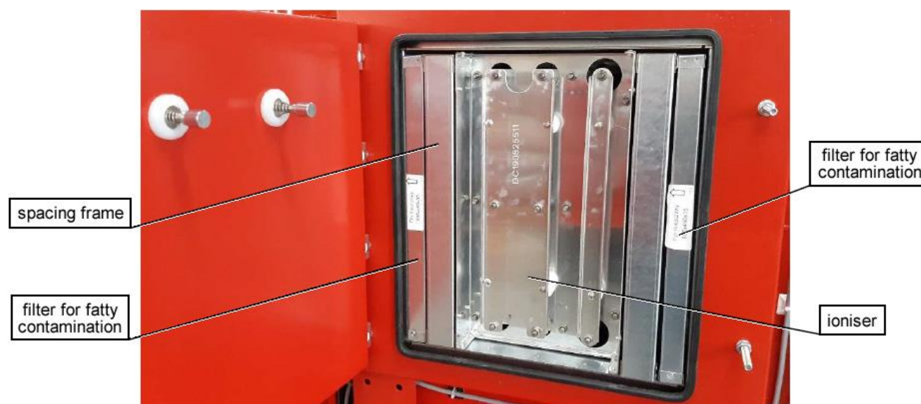
Photo No.2 – Filtration chamber – inside
