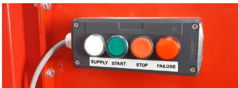
Photo No.5 – Control panel
