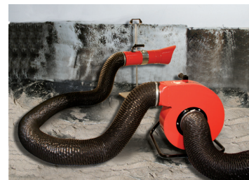
Extraction set used for drying the humid walls
