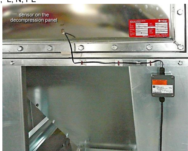
Fig. No.12 – Terminal box A3
