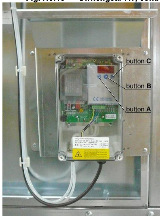
Fig. No.10 – Switchgear A1, control unit
