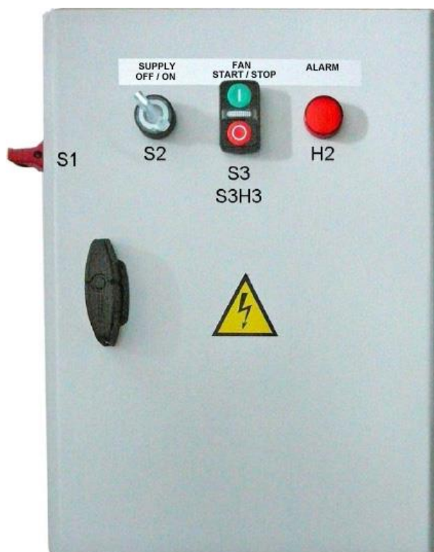
Fig. No.9 Switchgear A1
