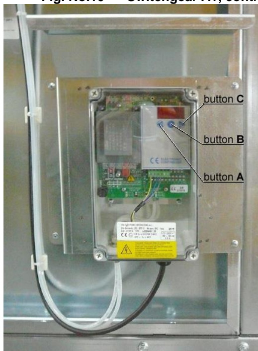
Fig. No.10 – Switchgear A1, control unit
