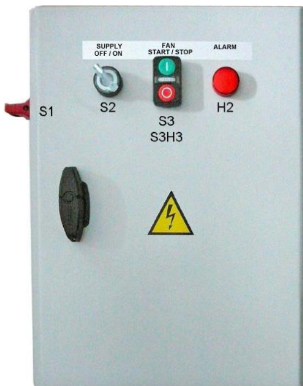
Fig. No.9 Switchgear A1
