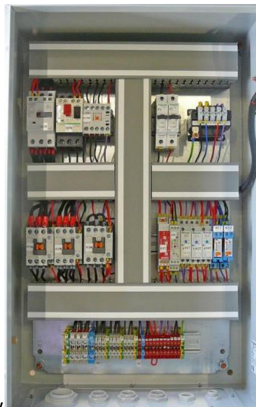
Fig. No.10 – Switchgear – internal view
