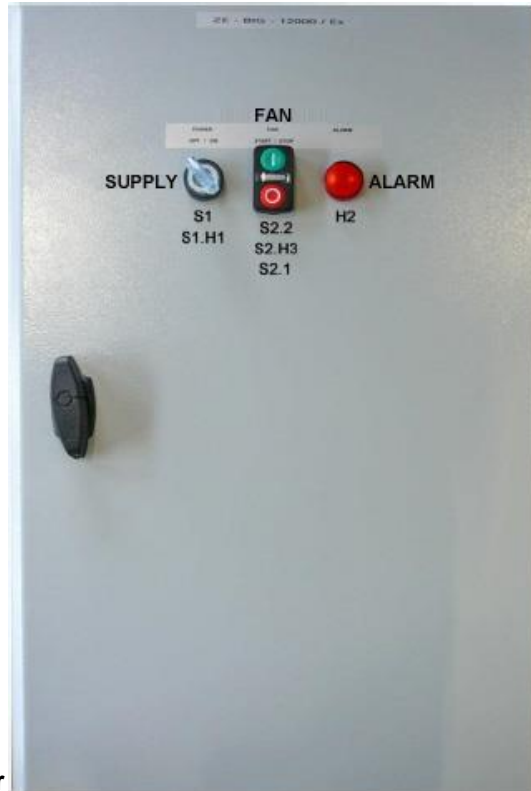
Fig. No.9 – Switchgear – Cover
