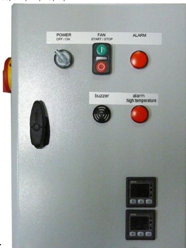
Fig. No.10 – Switchgear A1 – Cover
