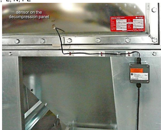
Fig. No.13 – Terminal box A3
