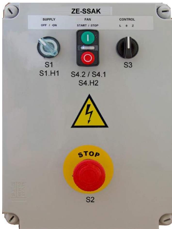
Fig. No.5 – ZE-SSAK control unit
