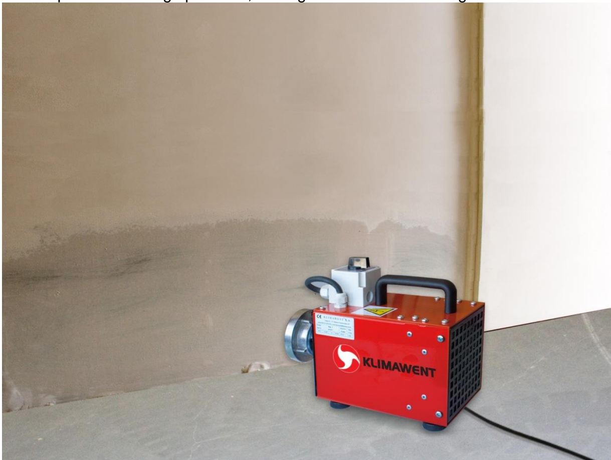
Photo No.3 – Drying up the walls
