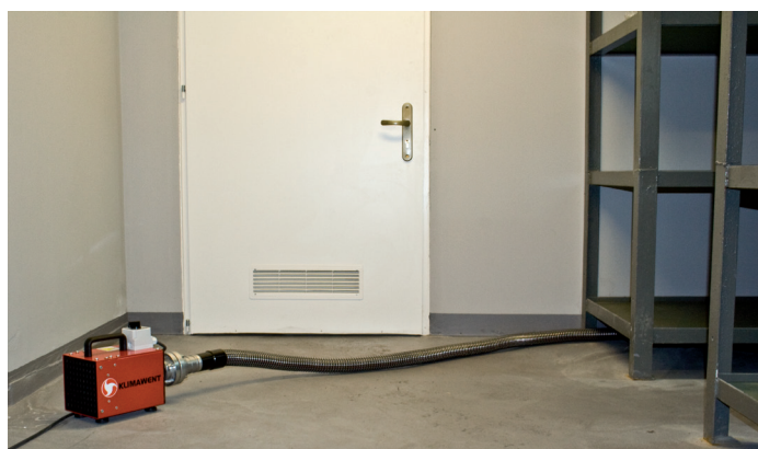
Drying of the hard-to-reach places through a hose
